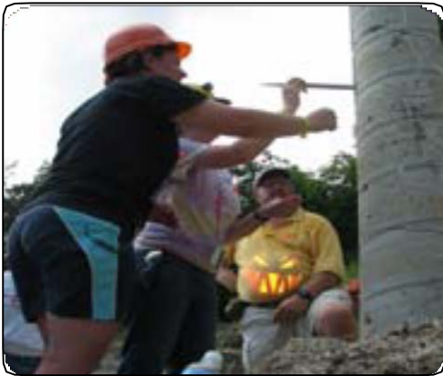
Loading of C4 for a demolition demonstration - 2005 Explosives Camp
